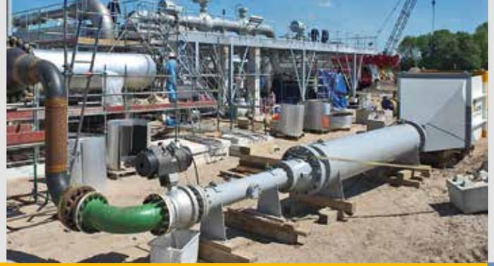
Air-blowing can be used as a safer, more environmentally friendly and cost-effective alternative to conventional cleaning and steam blowing. The purpose of air blowing is to remove loose scale and debris prior to start up using compressed air as the cleaning medium. The velocity of a large air mass through the pipeline will pick up any debris or loose scale left in the pipe. This method will guarantee the cleanliness of the compressor or turbine suction pipeline and prevent damage.
